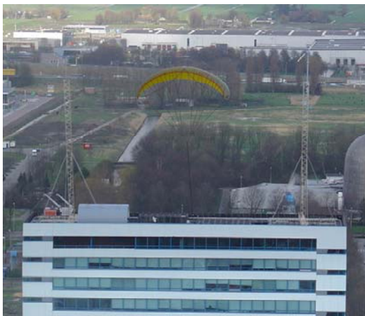
Figure 6: Kite laboratory to be built at the roof of the faculty building
