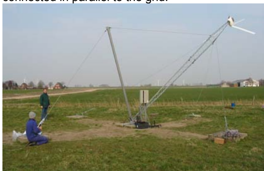
Fig. 4.3: Erection on the KWK test field
